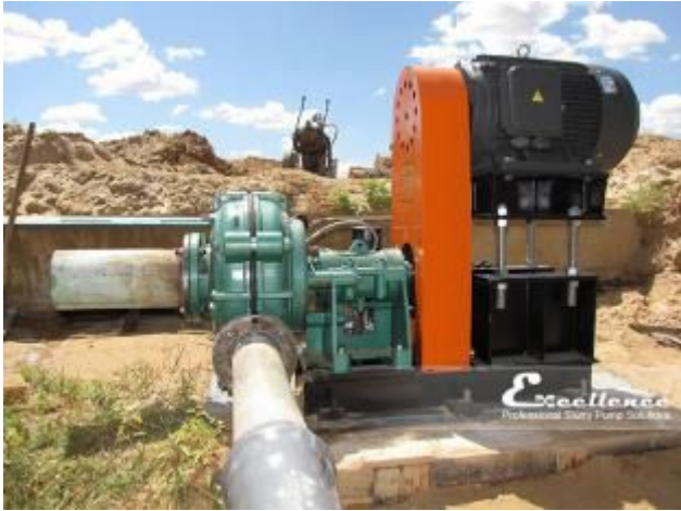
EHM-4D in Sand Excavation
